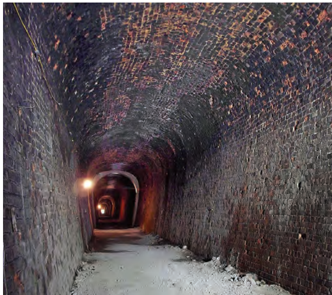
Looking west along the tunnel. Photo Ade Armishaw
